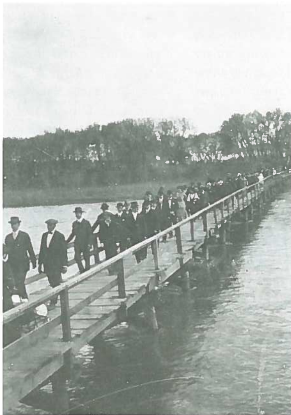
Above: Foot bridge to Assiniboine Park, c. 1912. This "temporary" foot bridge, which was installed every spring and removed before freeze-up in the fall, lasted until a permanent bridge was built in 1932. PAM N53.
