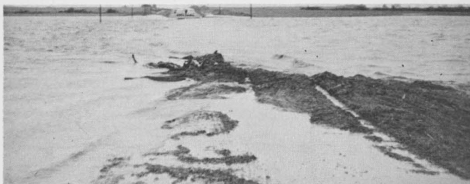
The flood of June 8, 1963 west of Cardale.
