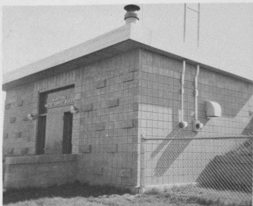
Oak River Water Treatment Plant. 1965.
