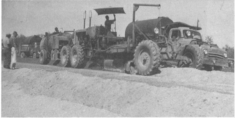
Building No. 50 Highway at Grimstead's corner.
