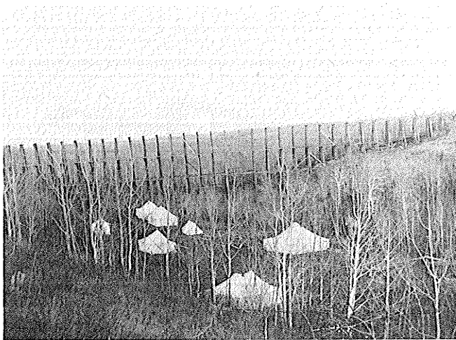
Camp at Thunder Creek Trestle. Rails were laid and used for several years. (Courtesy Manitoba Archives) 1909.
